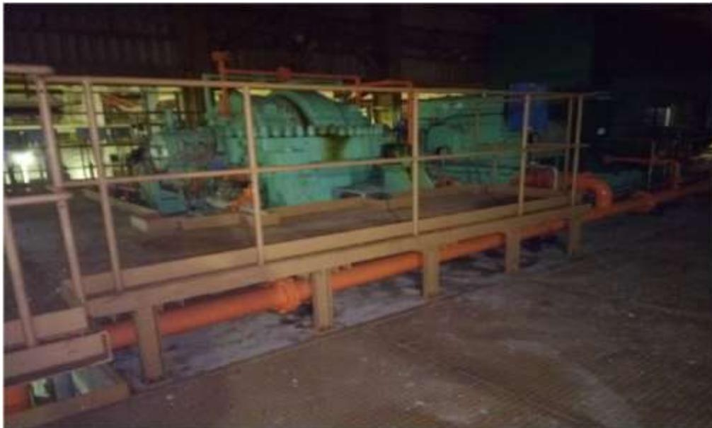
**Figure 8: Turbo-compressor of train 200**
