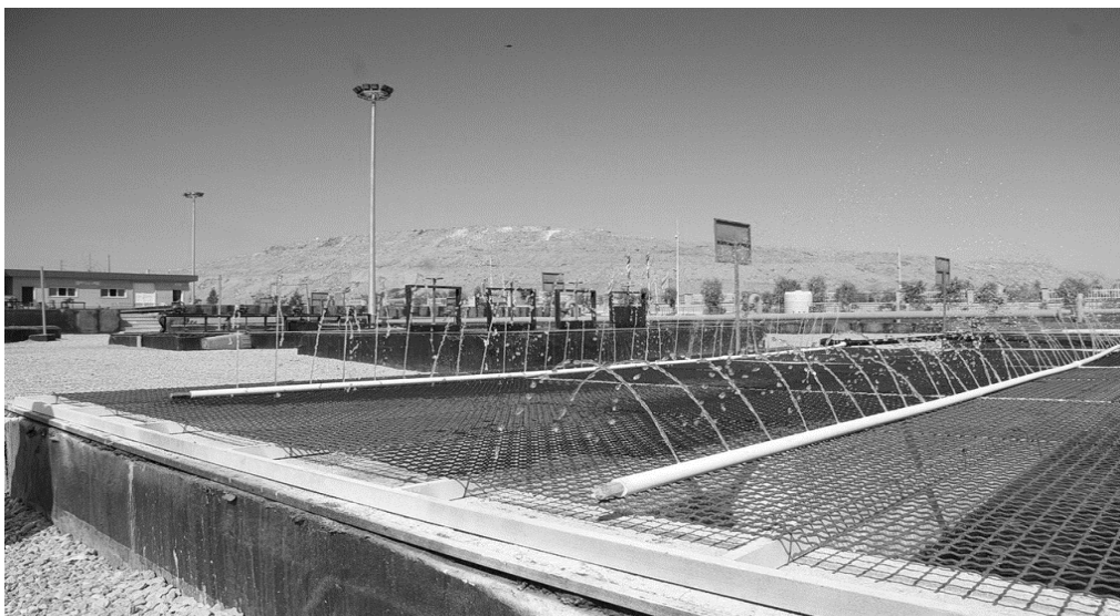
Fig.4. Treated leachate in TLTP
